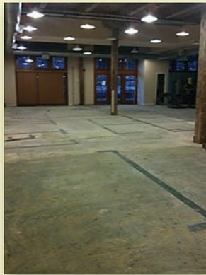
The slab in the 103-year-old building bore evidence of many past lives. It was of different colors, had cracks and heaves, and was covered in layers of mastic.
